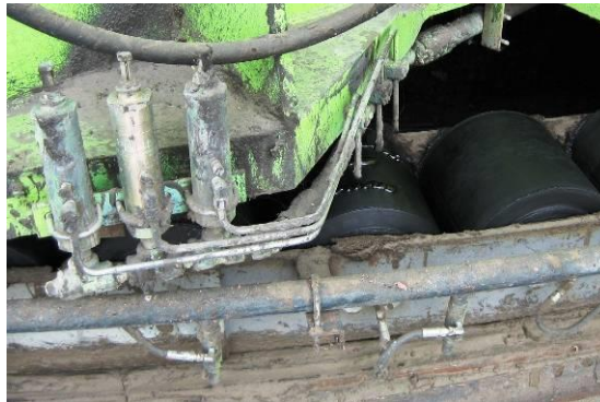
Dragline house rollers and rails
